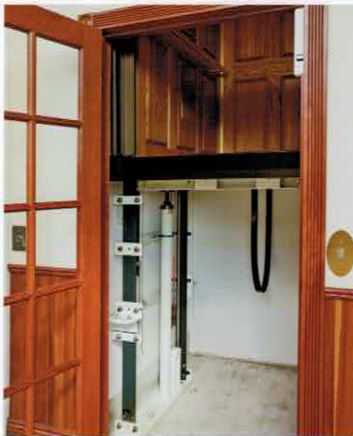
A close-up look at the mechanics of a residential elevator
